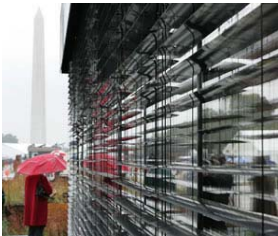
Automated external shading and krypton-filled glass help insulate Team Ontario/BC's solar-powered house. Photo by Stefano Paltera, courtesy of U.S. Department of Energy Solar Decathlon.
