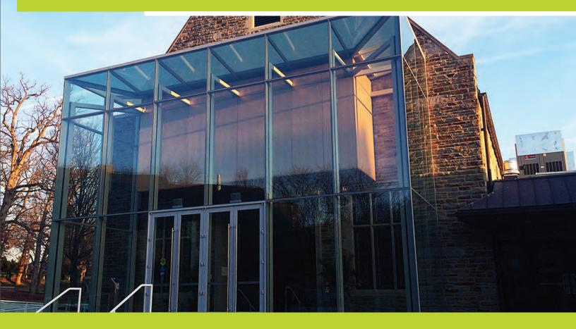
Solar Innovations, Inc. manufactured this four-sided structurally-glazed lean-to at the Friends School of Baltimore, MD. This type of glazing includes glass panels which are bonded to one another on all four sides, eliminating vertical framing members. The custom SI5200 structurally-glazed system includes a laminated roof and is used as the entrance to the institution. Visit solarinnovations.com to view more custom glazing projects.
