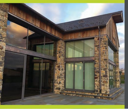
Solar Innovations, Inc. recently received the patent for its hybrid Marine Glazed System. This system combines the horizontal framing members of a stop glazing system with the vertical framing members of a marine glazing system to create the narrowest vertical sightlines on the market.
