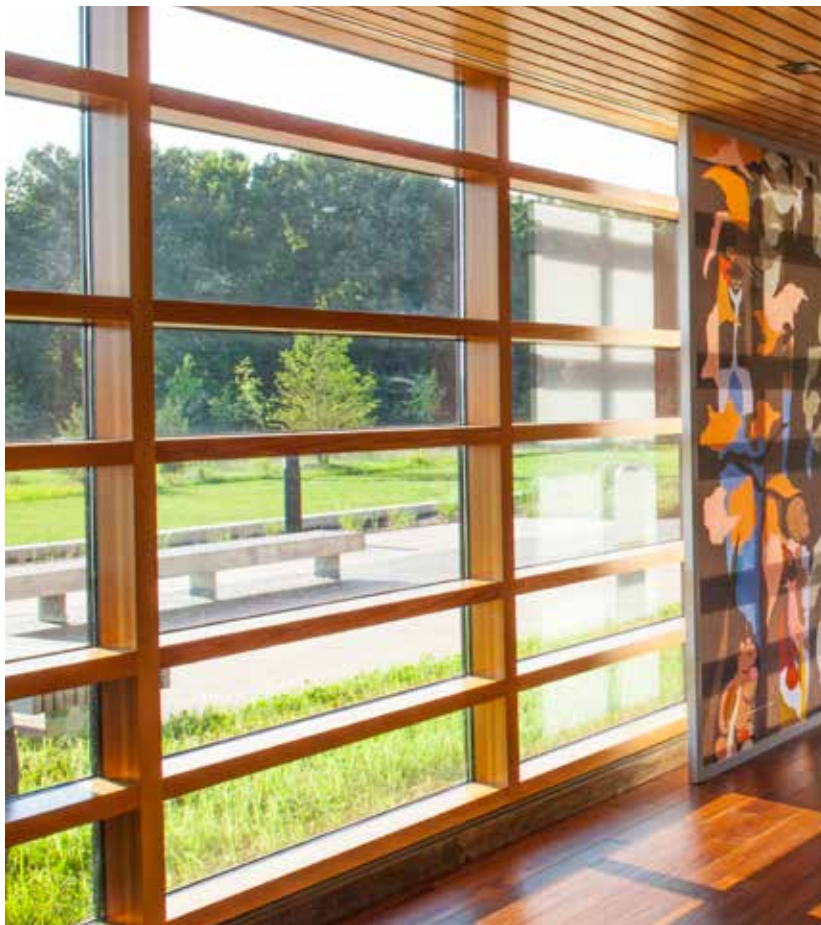
HARRIET TUBMAN VISITOR CENTER | CHURCH CREEK, MA Wood Curtain Wall
