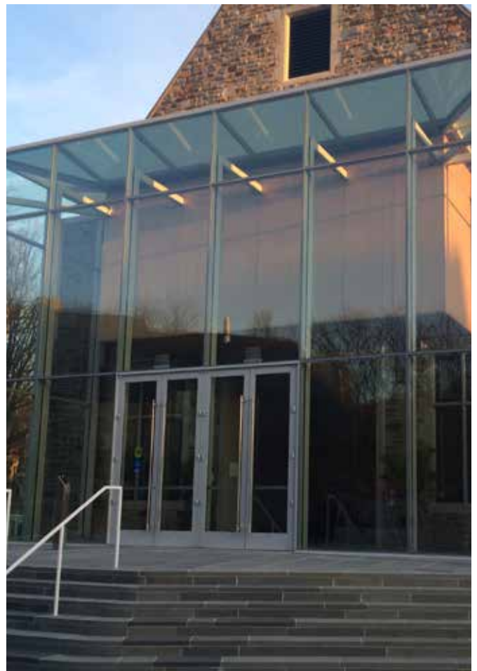
FRIENDS SCHOOL | BALTIMORE, MD Four-Sided Structurally Glazed Inverted Lean-To
