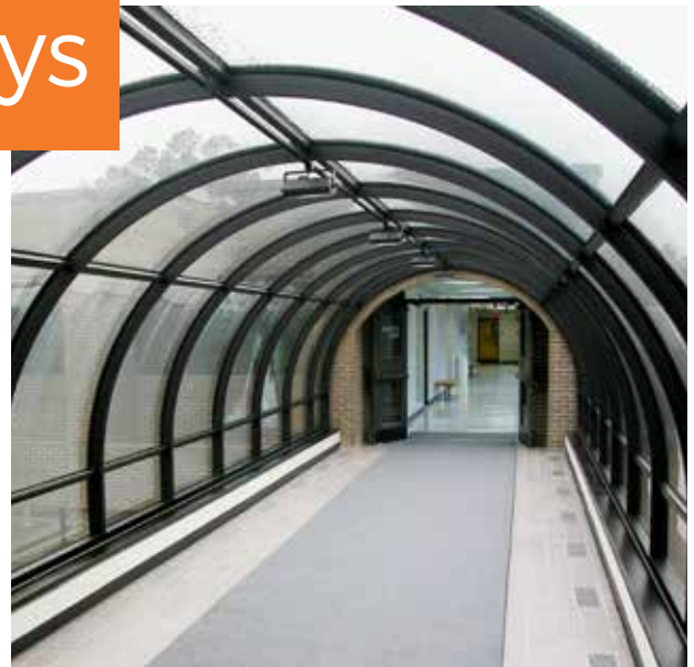
SAMPSON COMMUNITY COLLEGE | CLINTON, NC Barrel Vault Walkway
