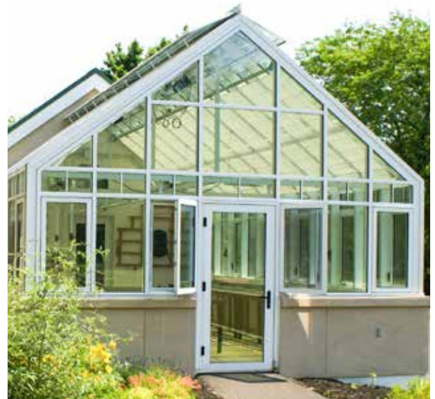
FOULKEWAYS COMMUNITY CENTER | GWYNEDD, PA Casement Windows
