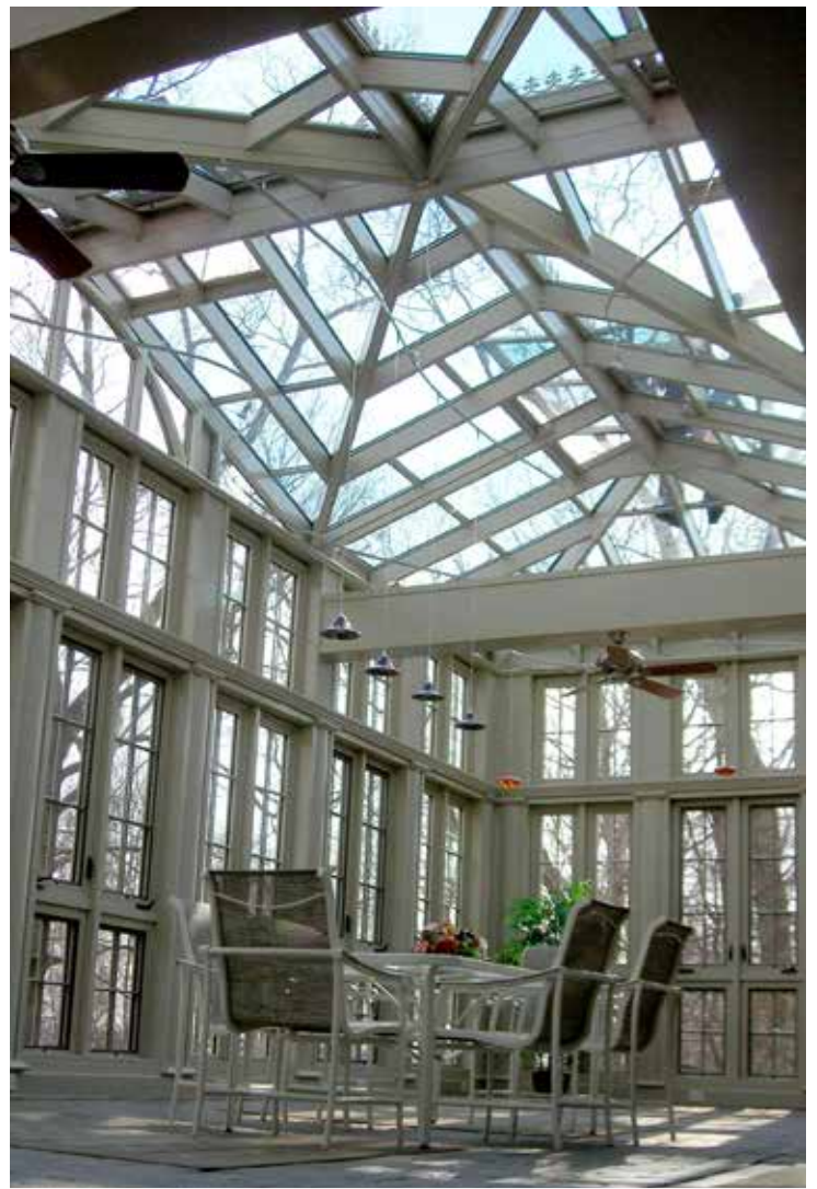
RESIDENCE | WARREN, NJ Straight Eave Double Pitch Conservatory with Hip End and Dormers
