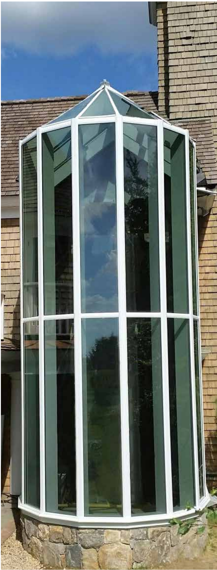
RESIDENCE | NORTH SALEM, NY 17-Sided Conservatory Nose
