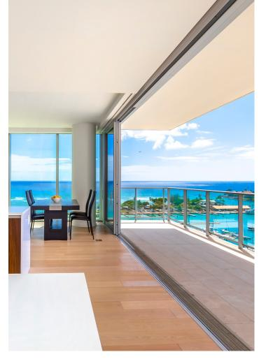
exterior of the door panels to blend the units seamlessly into the suites' contemporary design palette. To maximize the precious balcony space, finger grips were substituted for handles on the exterior of the doors, with the iconic Lift Slide handle implemented on the interior only. The Lift Slide Doors allow vacationers to enjoy the beautiful Hawaiian vista of Māmala Bay while providing the comfort and security of a high performance system.
