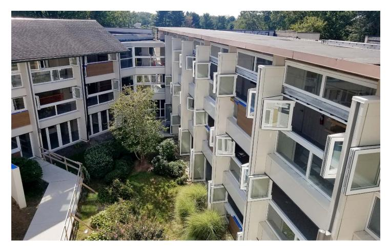
includes a covered walkway between the units that was exposed to the elements. To increase the energy performance of the buildings and give the residents an enclosed corridor to traverse during inclement weather, the architects planned to incorporate operable doors and windows in the walkways that not only would create a thermal barrier between the units and the outdoors, but also allow fresh air to circulate when the weather is nice.
