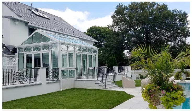
SERIES SI5204 Straight-Eave Double-Pitch Conservatory with 2 Gable Ends SI3351 G2 Folding Glass Wall and Window FINISH White GLAZING 1/4" LoE 366 tempered over 1/4" clear tempered with .060 PVB interlayer (Argon filled) GLASS SQUARE FT. 1002 sq. ft.
