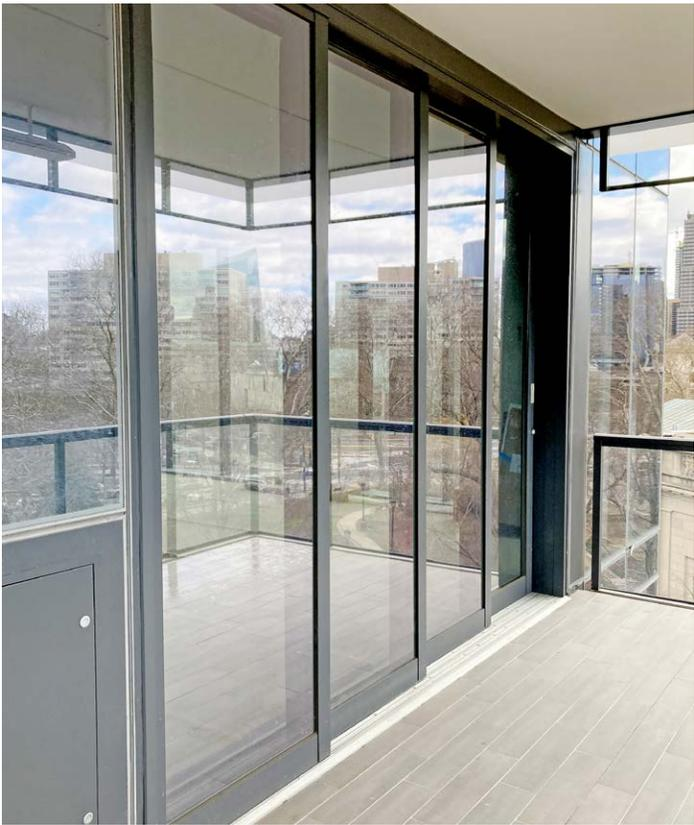
To address the large outside corner openings on the street and penthouse levels, six-panel, no-corner-post units (OXX-XXO configuration) were selected. In both cases, this configuration expanded the indoor entertainment space to large outdoor patios, blurring the line between interior and exterior spaces. And for ease of use, each unit was motorized for effortless operation.
