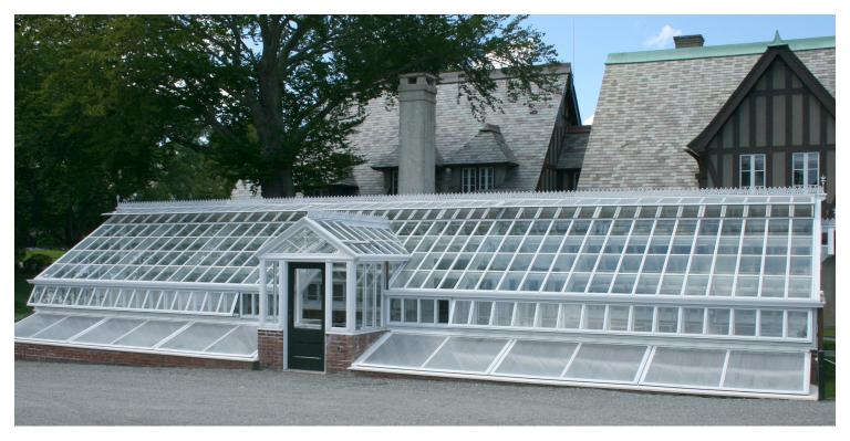
SI5000R series is a modern, thermally enhanced glazing system intended to replicate the delicate structures of the past. The glazing bars have a historic shape when compared to a flat faced modern bar. The glazing is insulated and tempered compared to single pane and only annealed. Wheels can be created to turn the ventilation as in older greenhouses in replacement of modern electric motors.
