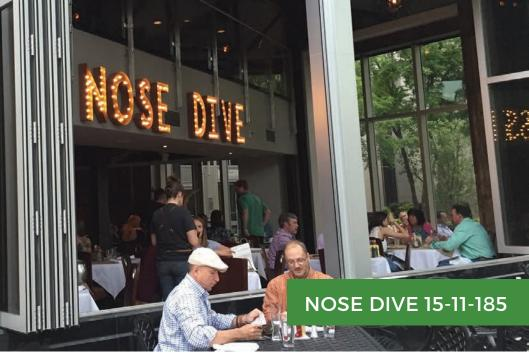
Nose Dive features two 12' tall center pivot folding glass window systems utilizing center hung trolleys on each panel.
